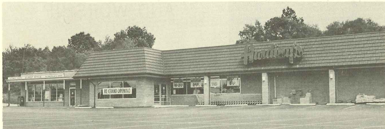
Located at the north city limits are a newly modernized grocery store and the U.S. Post Office.
