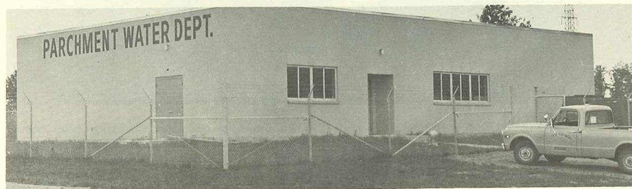
The new City Water Department with it's iron removal plant was constructed in 1974 at a cost of a half million dollars.
